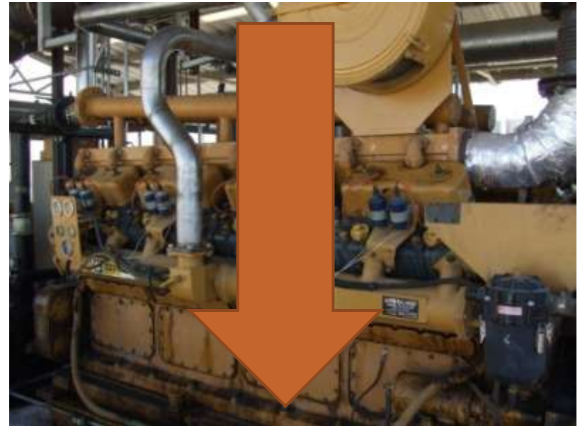
Gas Engine Low investment cost Low maintainance Lower efficiency
